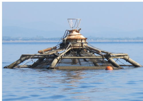
Sadco Shelf cage – rigid frame, submersible
