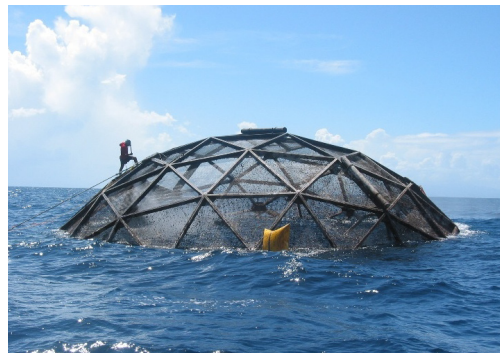
Aquapod – geodesic sphere, submersible
