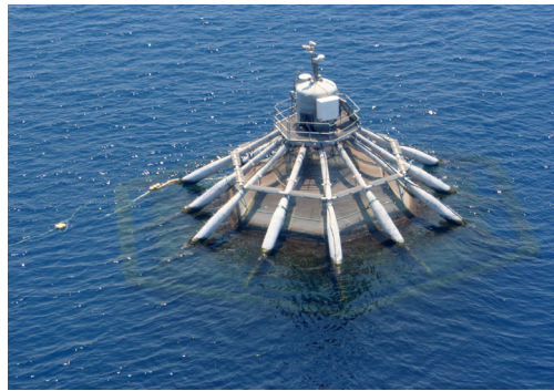
FarmOcean cage – semi-submersible, reduced surface exposure
